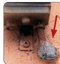
Corrugated pipe entry protection
