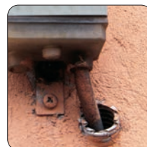
Corrugated pipe entry protection
