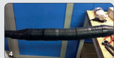
4 The joint is completed and can be used immediately.
